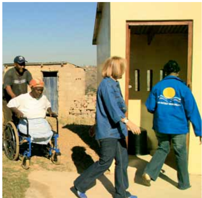
VIP toilets for the physically challenged
